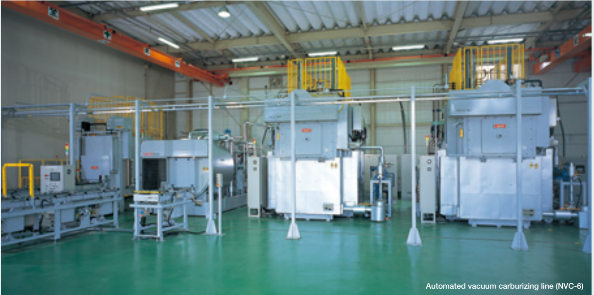
Automated vacuum carburizing line (NVC-6)
